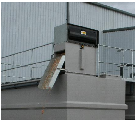
Model 600 Auto-screen removing vegetable Solids prior to biological treatment of the Effluent.
